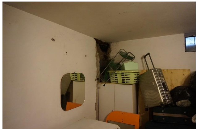
Piano seminterrato – Cantina
