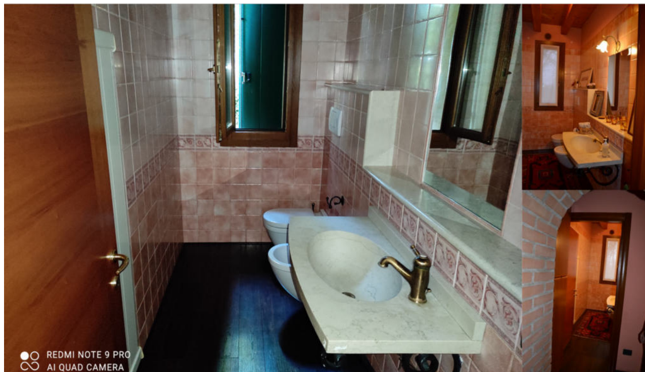
Figure 35-36-37- BAGNO AL PIANO TERRA;
