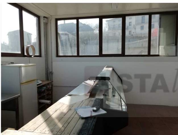
Locale piano terra
