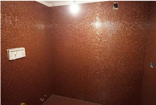
Piano interrato – Bagno
