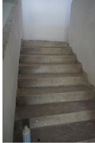
Piano terra – Scala interna
