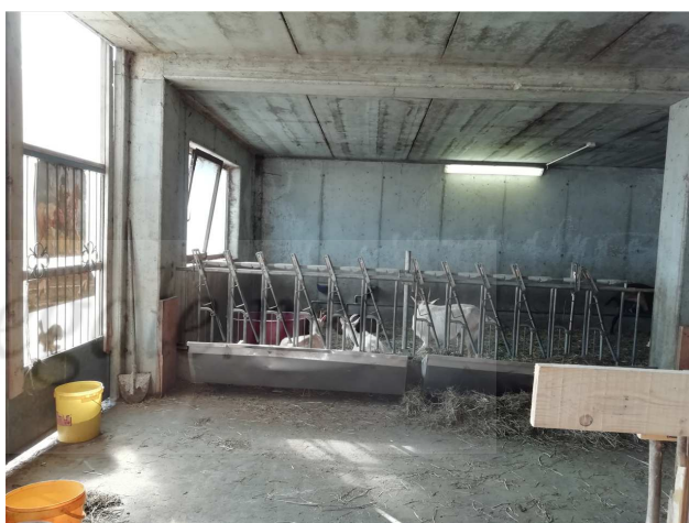
Vista stalla – piano seminterrato
