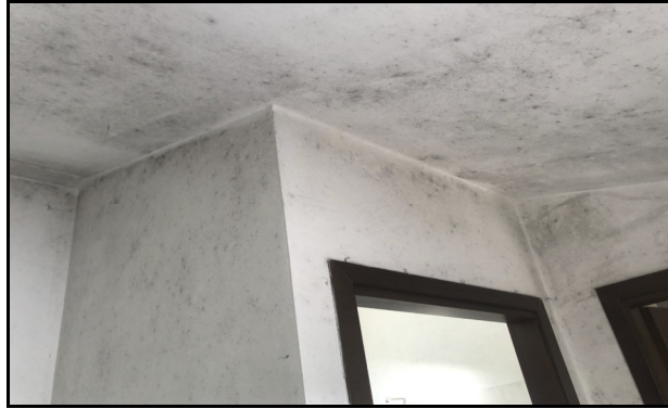
SOFFITTI PIANO III^
