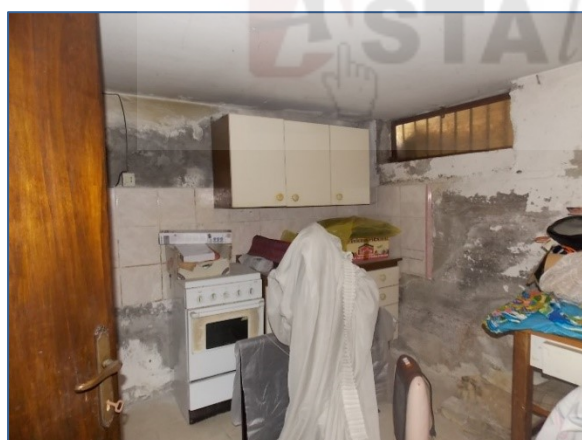
Piano seminterrato cantina
