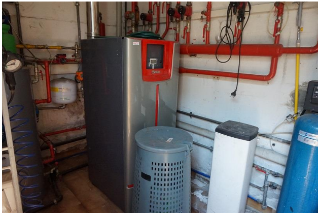
Piano terra – Locale C.T.
