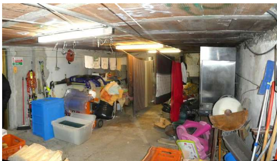
43. – locale Lavanderia – piano Interrato
