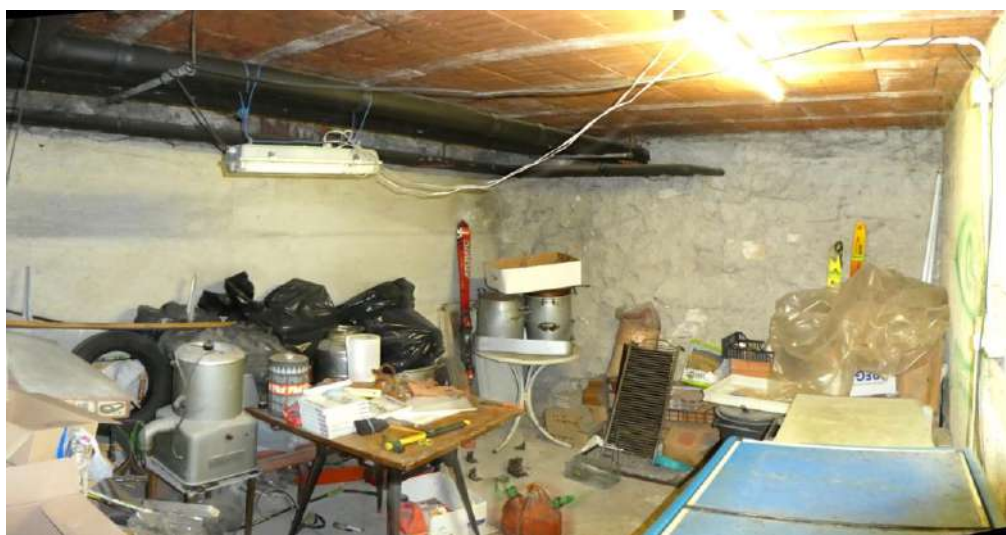
42. – locale Cantina – piano Interrato
