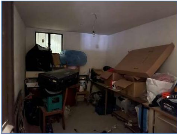
11. Piano seminterrato - Cantina
